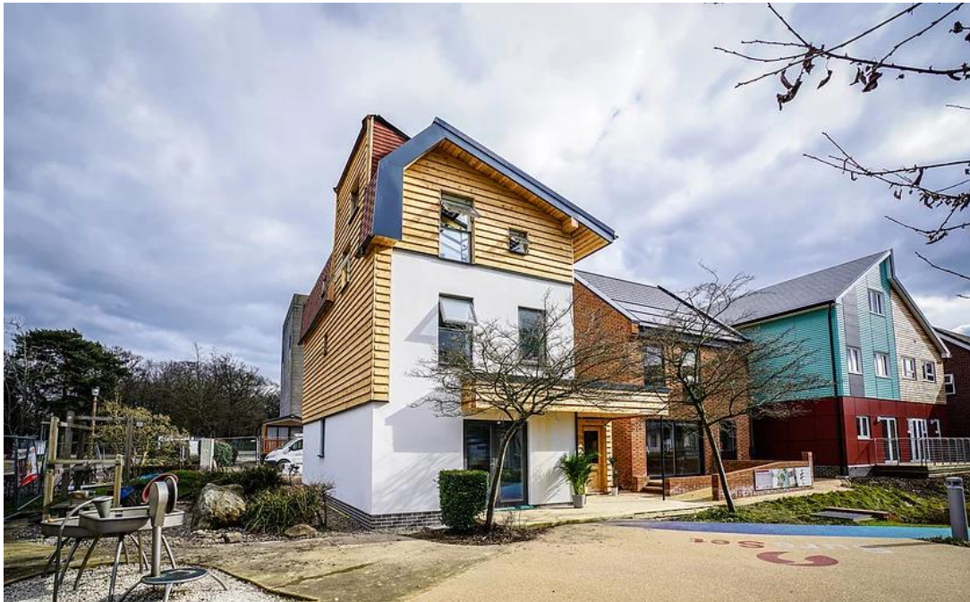
Figure 3 The Zero Bills Home at Building Research Establishment - achieves net negative carbon through efficient design, a heat pump, solar PV plus battery
